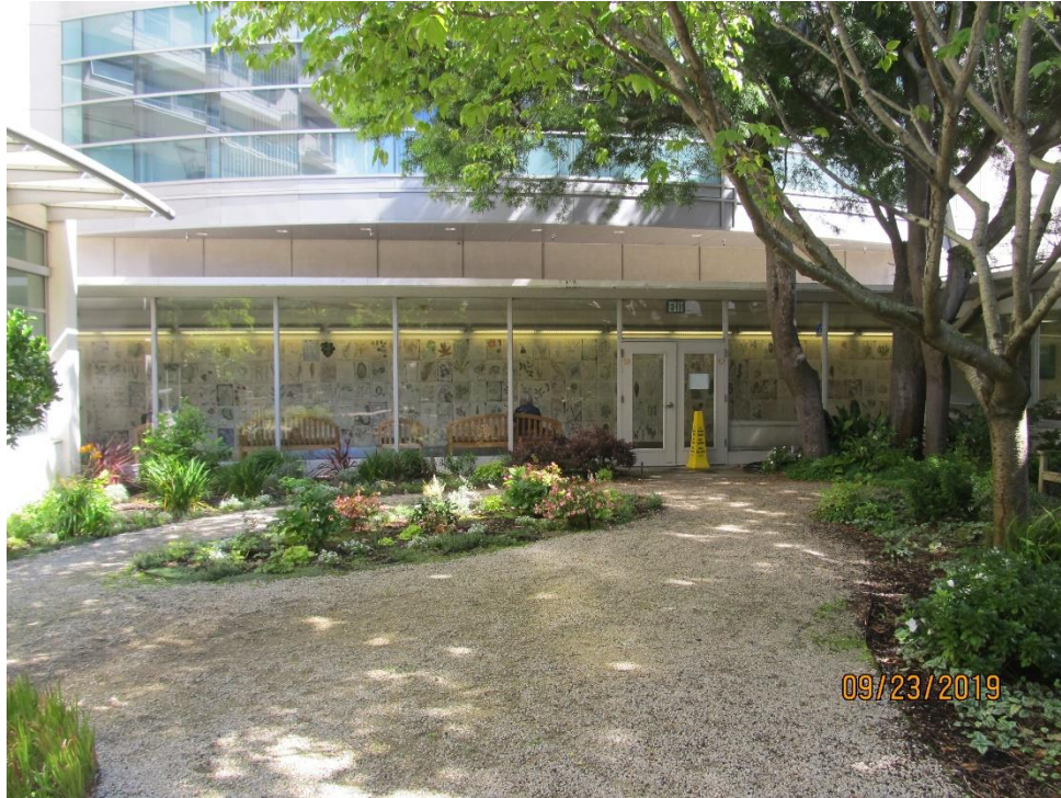
West elevation of the Administration Building (looking east)
