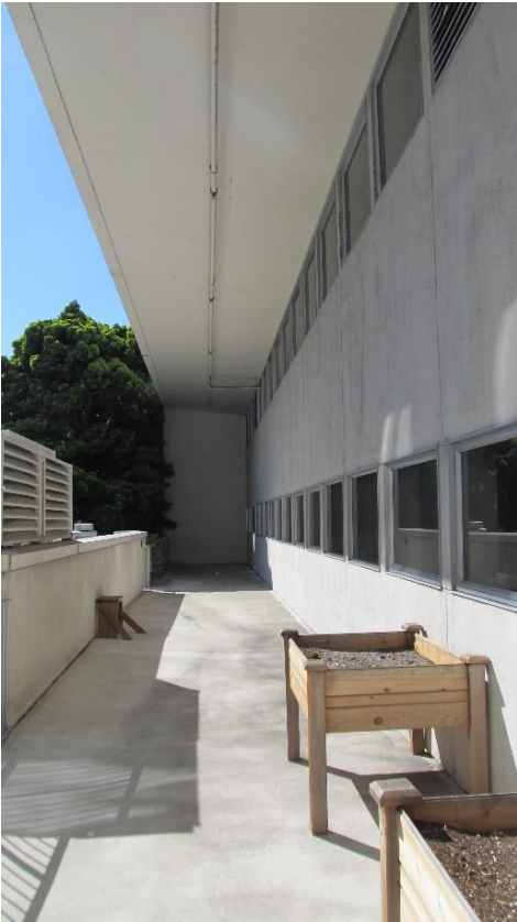
Covered balcony at second floor (looking west)
