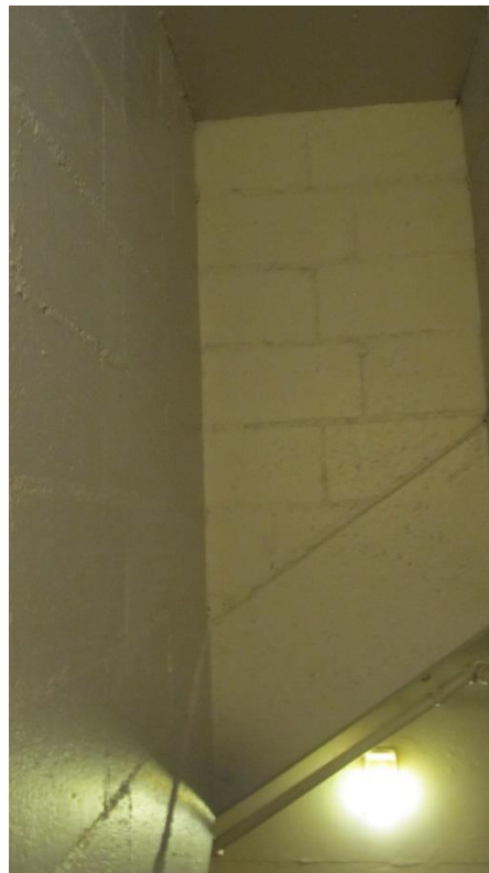
CMU walls above at elevator penthouse
