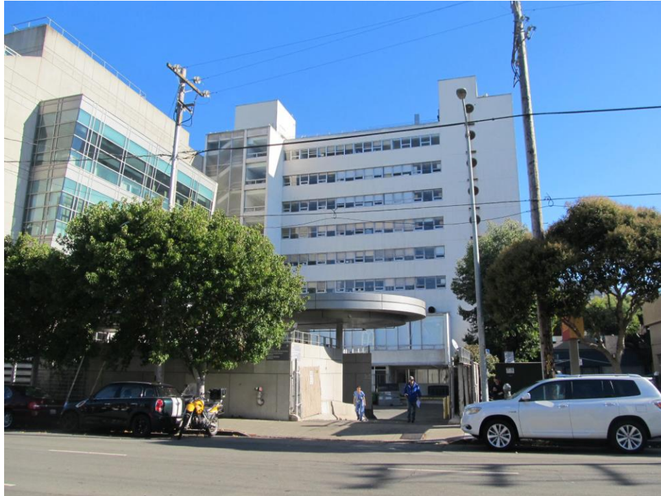
North elevation (looking south)
