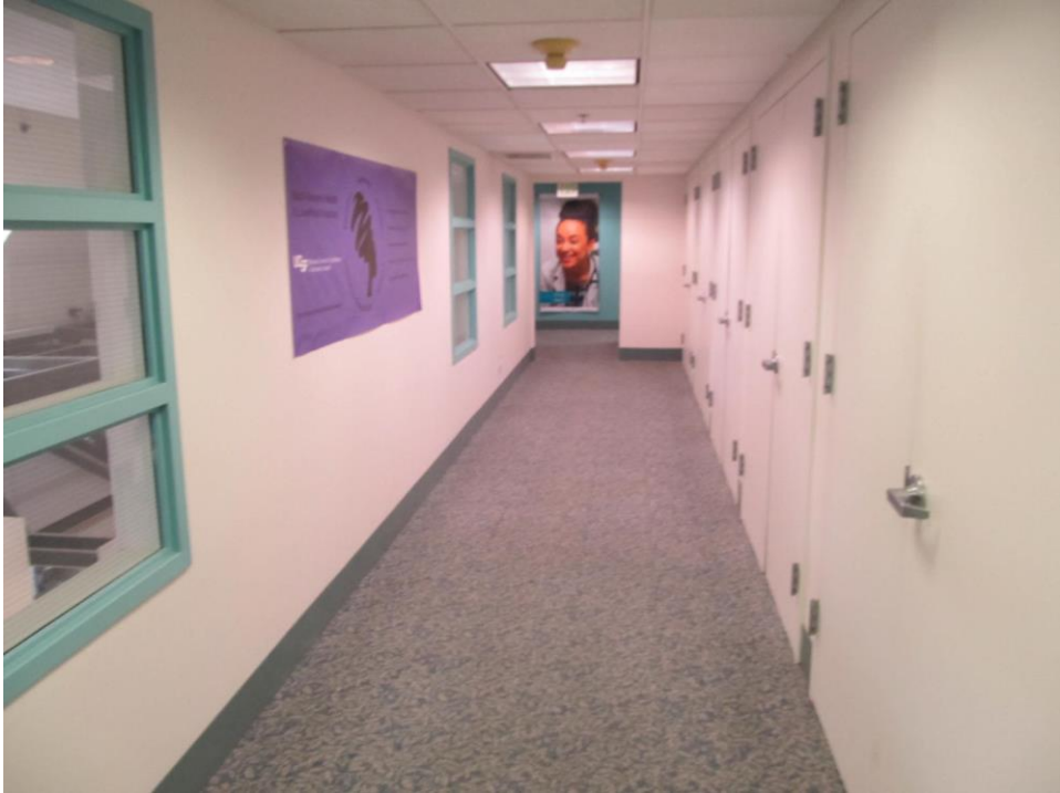
Hallway at mezzanine (looking west)
