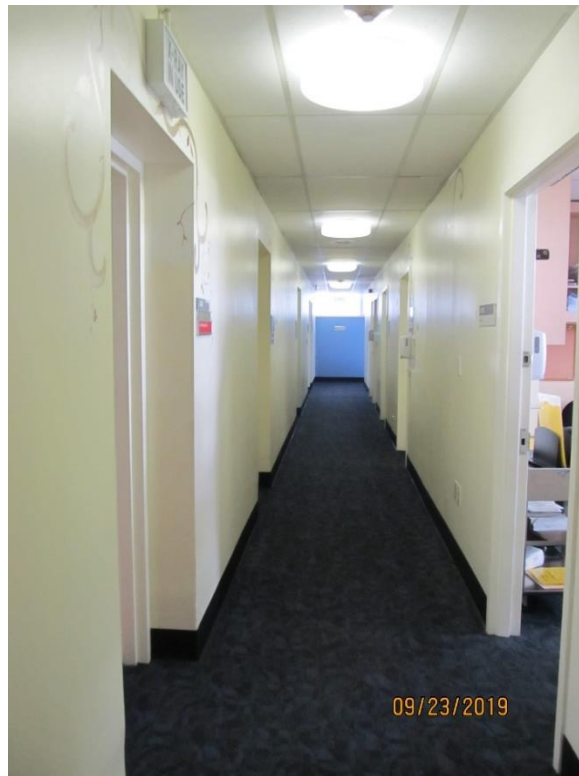
Corridor in the Administration Building. The concrete shear wall is on the left (looking west)
