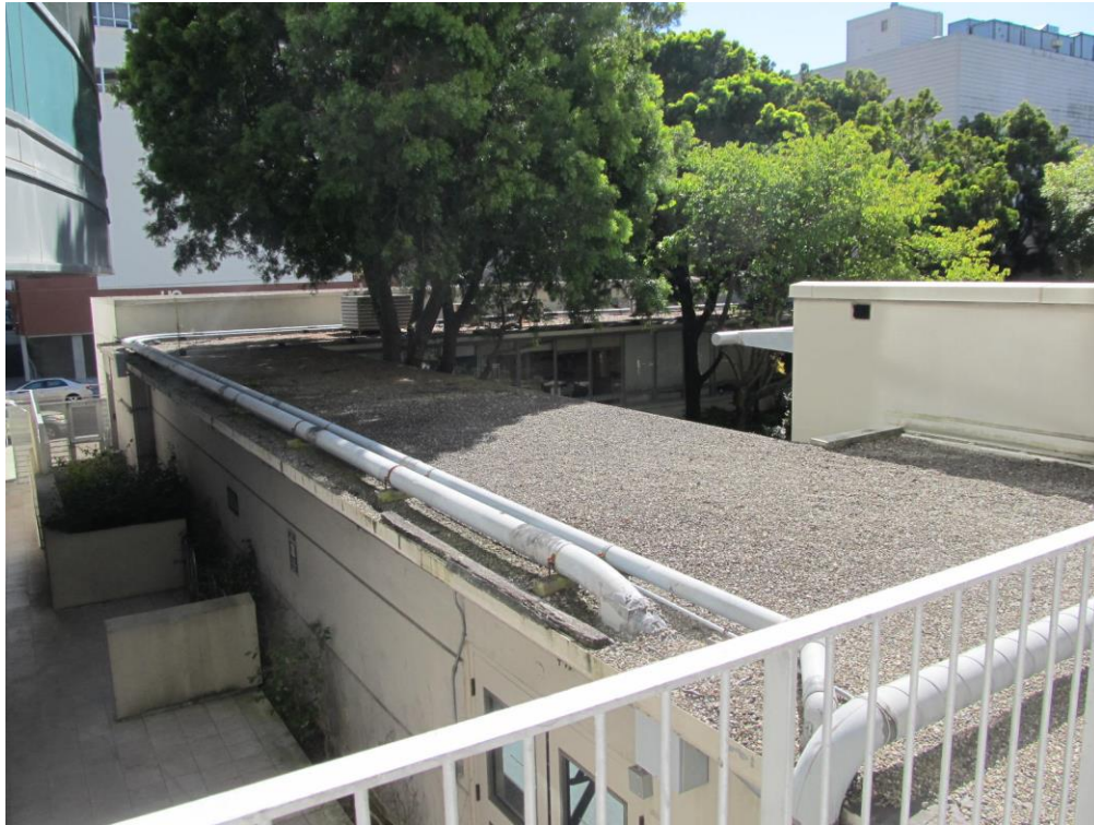
Tar-and-gravel roofing at the Administration Building (looking southwest)
