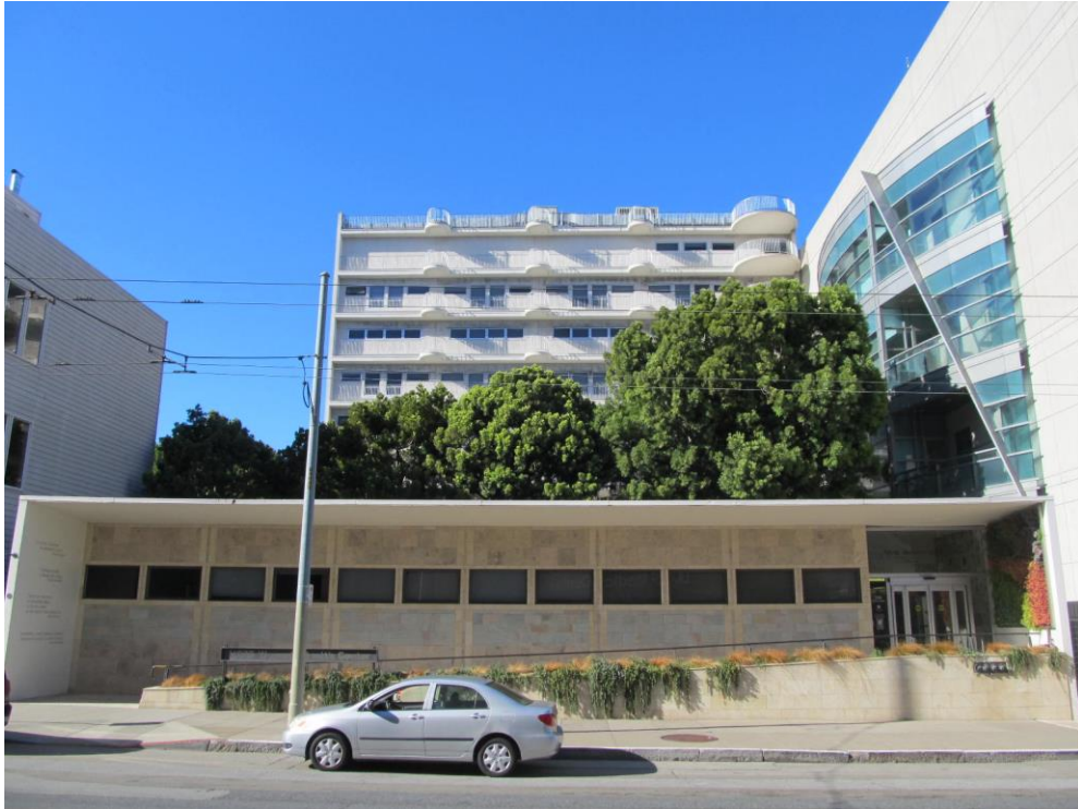
South elevation. Administration Building in the foreground and Main Tower in the background (looking north)
