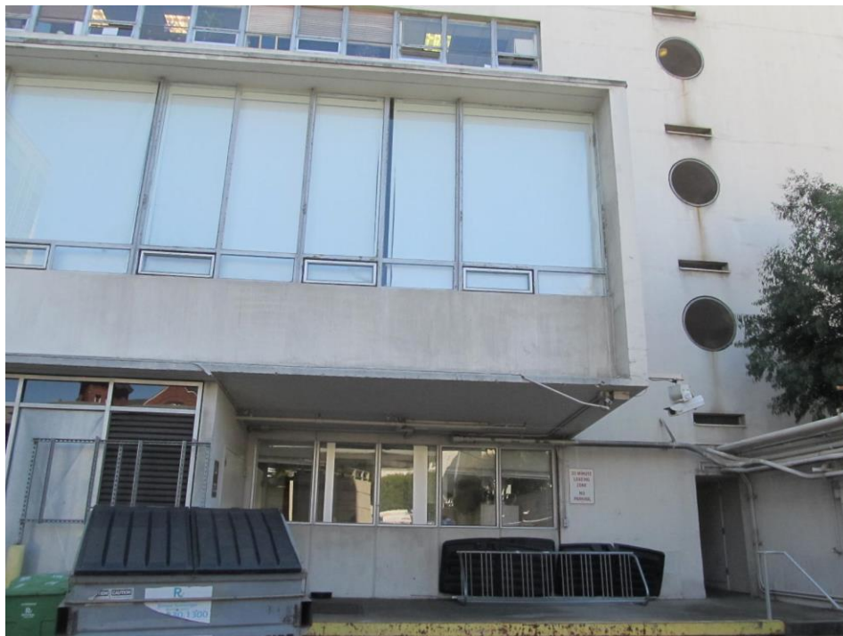
Discontinuous wall at north elevation (looking south)
